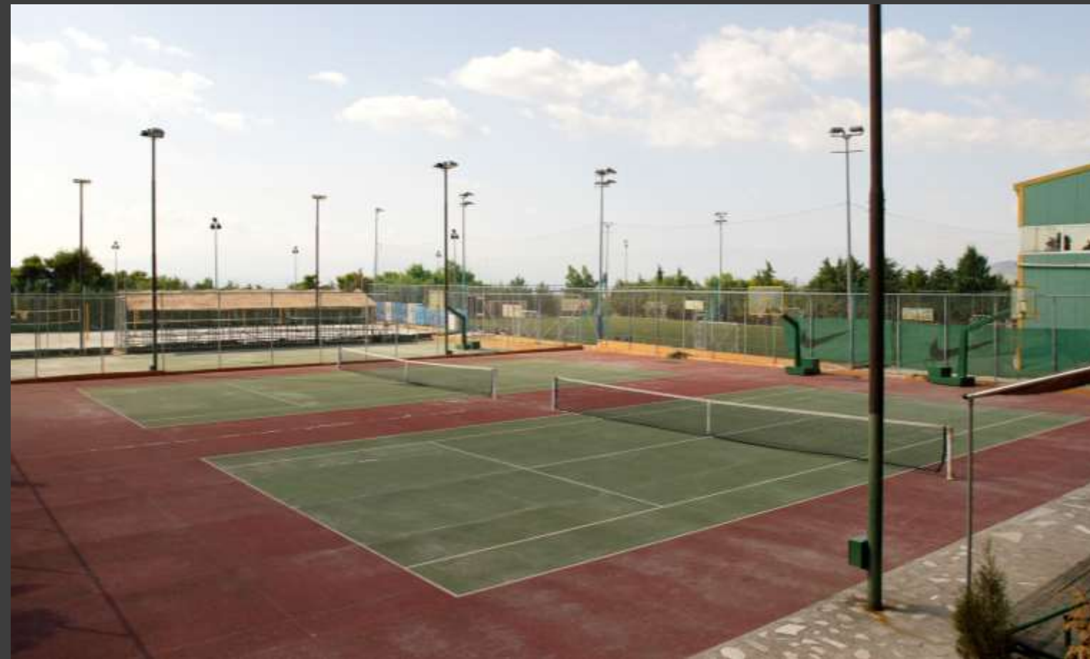
3 tennis courts (Quick surface)
